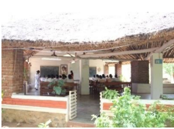
Old school building
